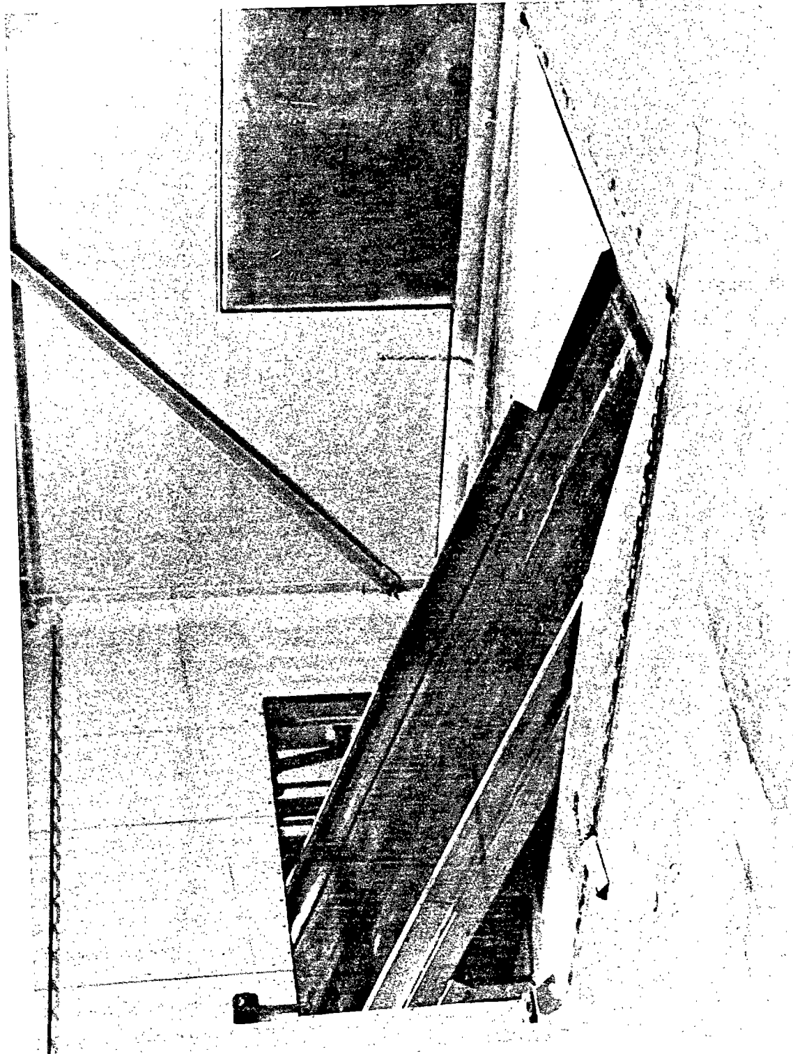
FIGURE 4 - FEED CONVEYOR IN FEED ROOM FOR CONTINUOUS FEED
